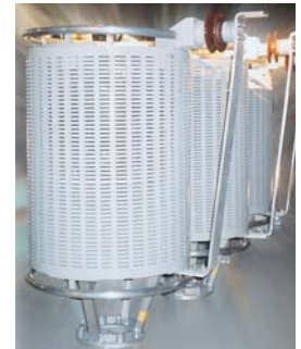
Vertical pedestal A line traps featuring line connection at the top
