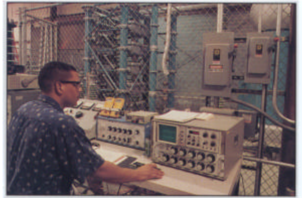
1,500,000 V Impulse Generator
